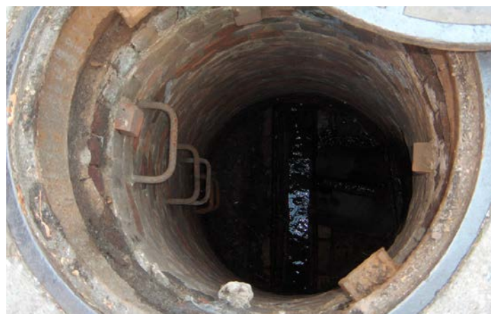
Sewer entry point
