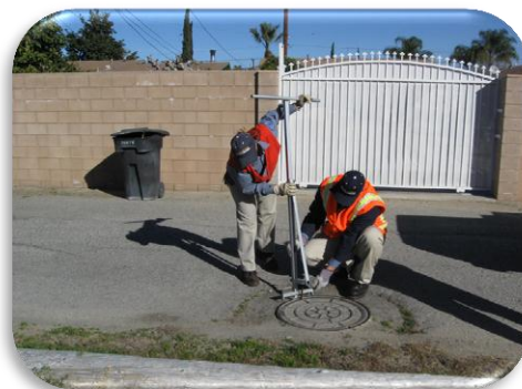
Vector Control Technicians conducting a sewer survey.
