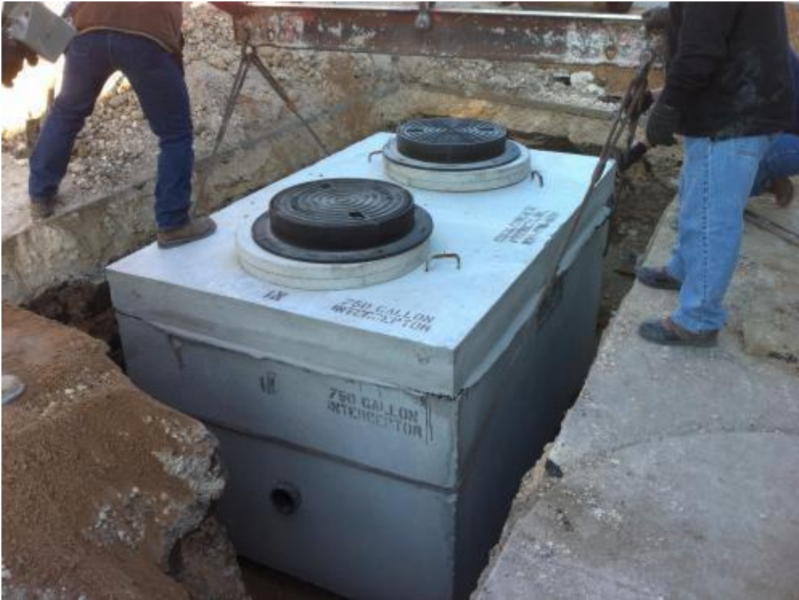
Figure 9: Grease Interceptor
