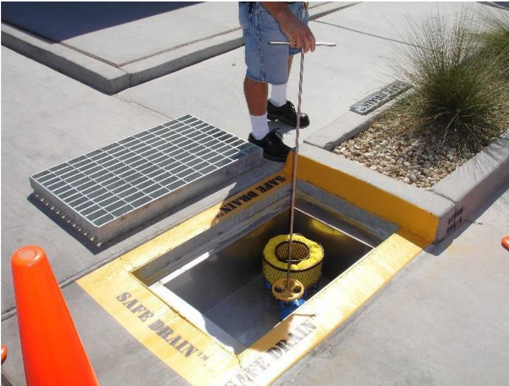
Figure 12: Stormwater Best Management Practice (BMP)
